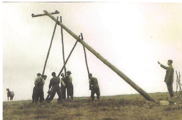
Erecting poles in 1950s
