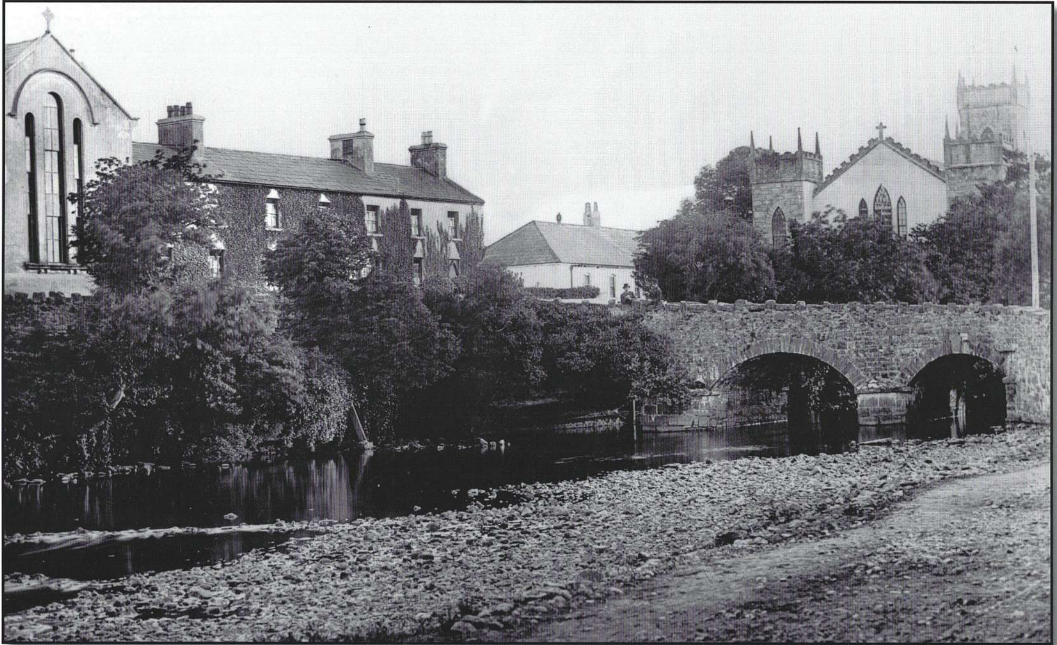
The Bridge and Convent of Mercy (1857-2013) with the Catholic Church in the back ground. The Sisters of Mercy were invited to Oughterard by Rev. Fr. Kavanagh P.P. and replaced The Faithful Companions of Jesus (1843-1846). Four sisters took possession of a small house near the church which was provided rent free. Funds were scarce and classes were held in out offices but by 1863 there were 345 children on the school roll. The present Primary School building dates back to C 1888.
