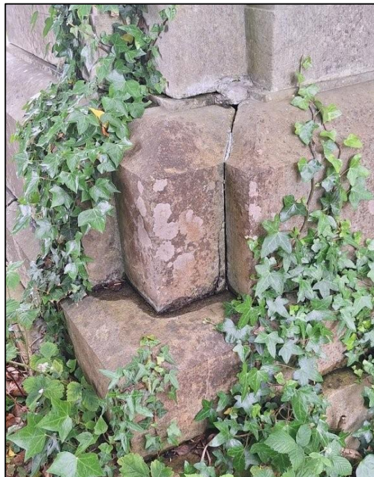
Plate 40 Memorial requires minor repairs to reinstate capping. Base of missing cross can be found on the ground ready for reinstallation. <maintenance to the railings is advised. This work is incidental to phase1 proposals
