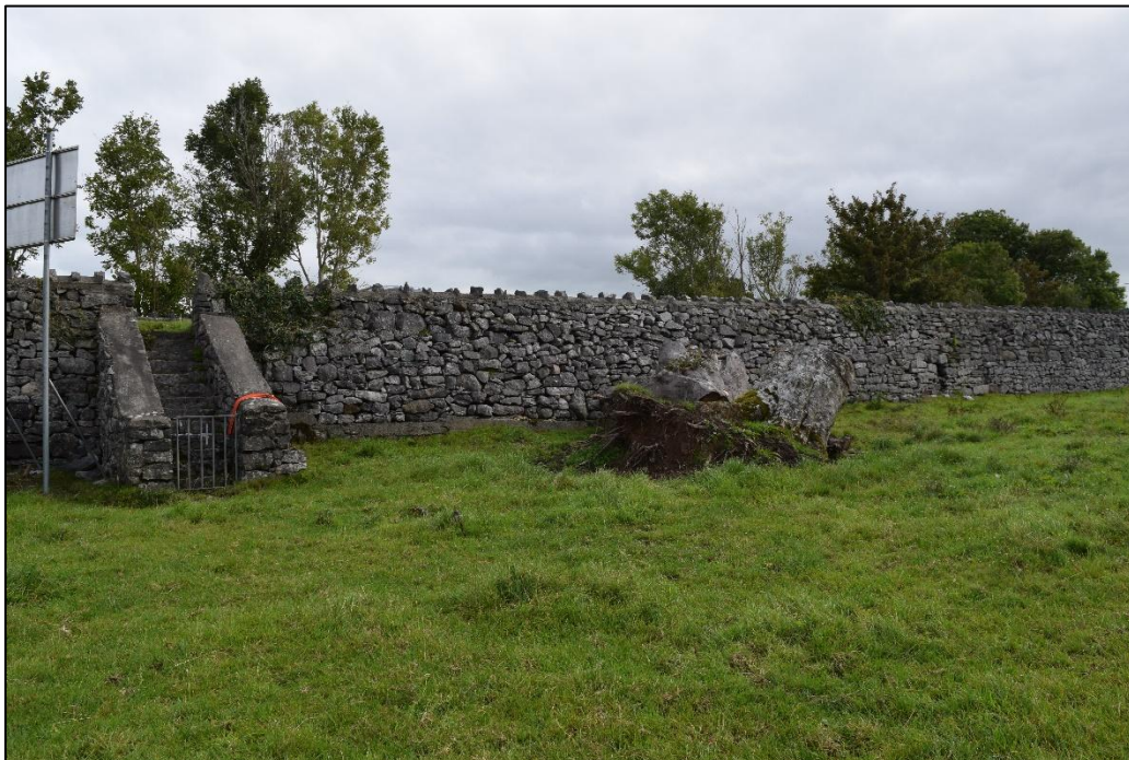
Plate 44 Access to the well is formalised with steps and a pedestrian gate
