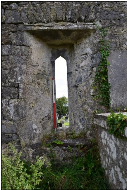
Plate 22 East elevation, interior of slightly off-centre ogee-headed light suggests a fourteenth century date however this may be set into earlier fabric as a later alteration. Note later remining interior lime plaster.
