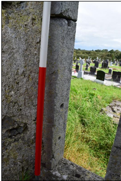
Plate 26: East elevation, interior; ogee-headed window opening, sockets for window joinery (transoms) visible.
