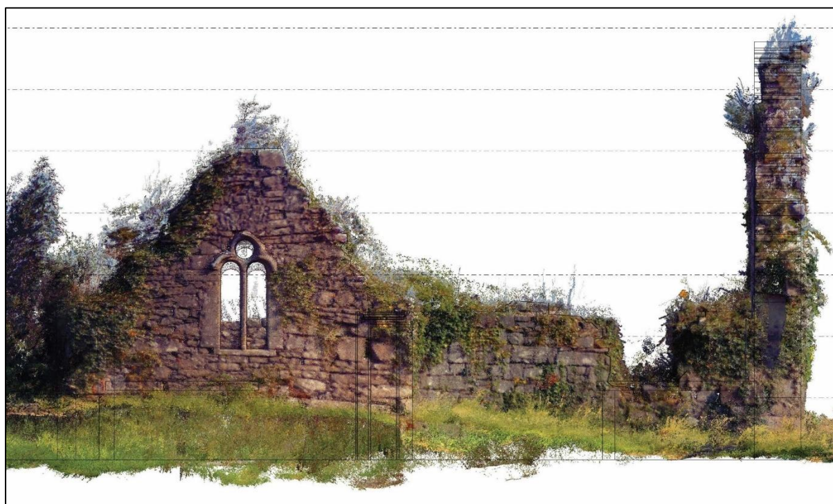
Sketch H: showing east elevation of South Transept. Vegetation treatment to be completed in Phase 1 and masonry works in Phase 2.
