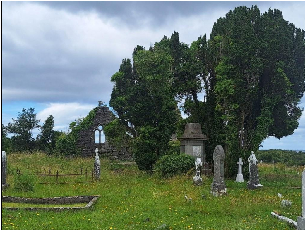
Plate 3 Approach showing south transept gable access is difficult and will require clearing
