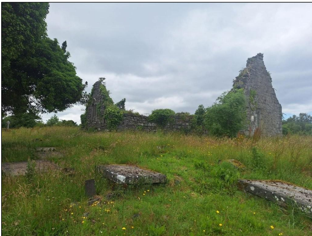
Plate 4 View of east gable (right) and south transept (left), facing northwest.
