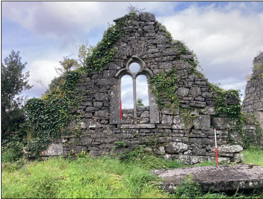
Plate 7 View of the south transept of the south elevation
