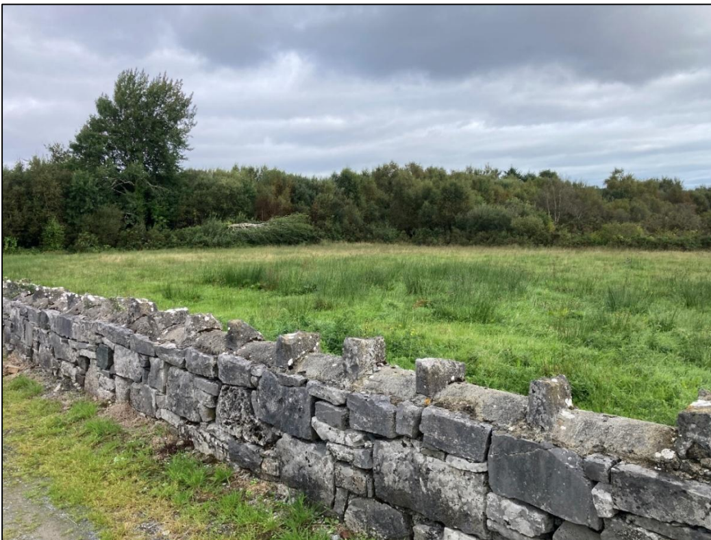
Plate 2: Northern boundary wall; dry-stone wall with cow-and-calf mortared coping
