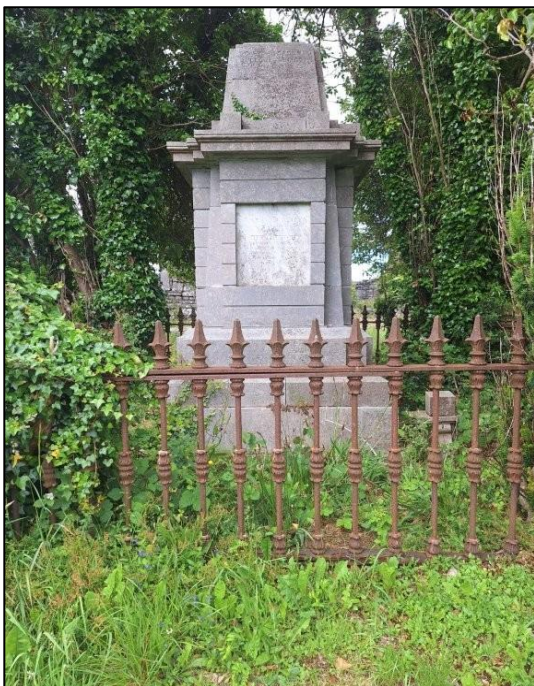
Plate 40 Memorial requires minor repairs to reinstate capping. Base of missing cross can be found on the ground ready for reinstallation. <maintenance to the railings is advised. This work is incidental to phase1 proposals
