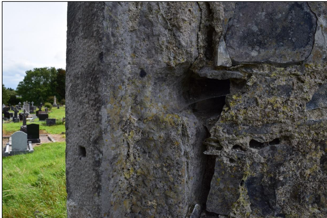
Plate 27: East elevation, ogee-headed window reveal with sockets for window joinery and large socket possibly for securing a window shutter closed.
