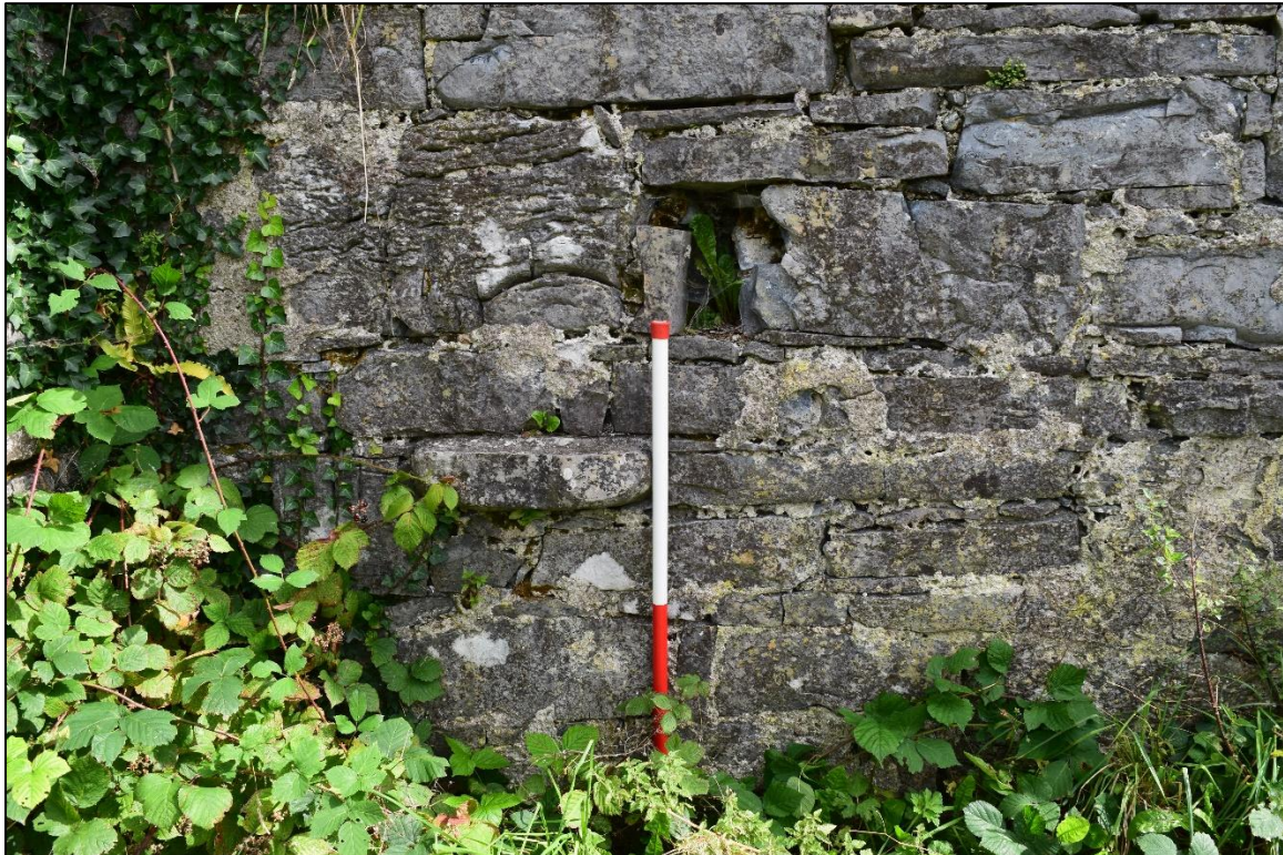
Plate 25: East elevation, interior: north side of window an opening is present and low masonry projection with small socket presumably part of interior liturgical scheme.
