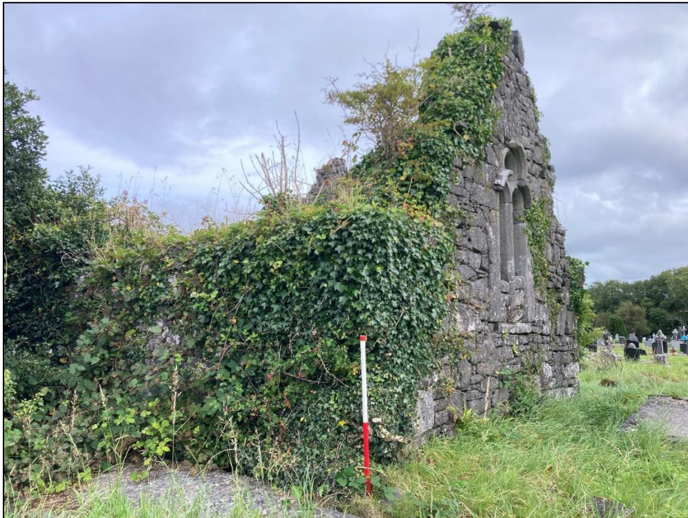
Plate 37: West elevation of south transept
