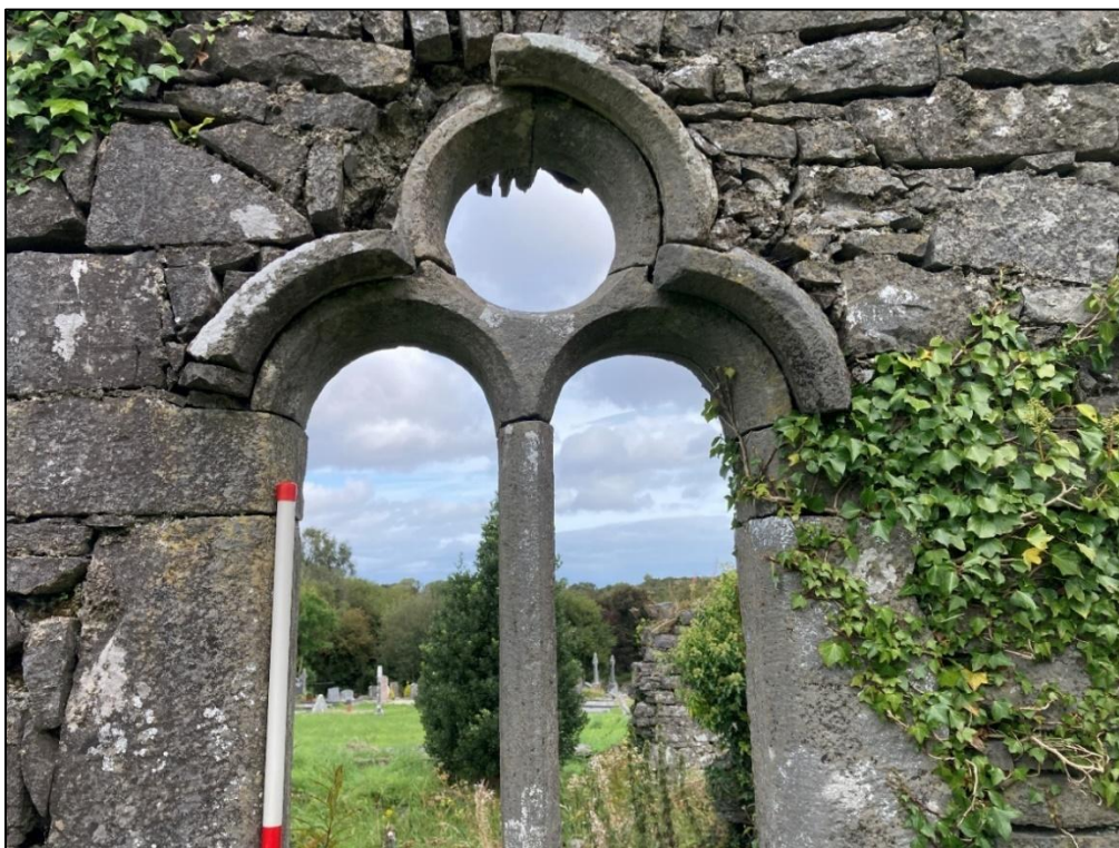
Plate 8 Twin light, round-headed window with circular oversight and tri-partite carved limestone hood-moulding in the south elevation.
