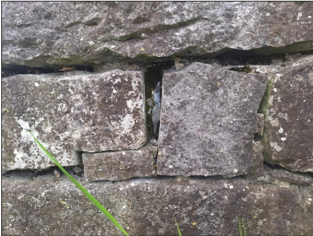
Plate 24 Tying stone in cyclopic style masonry in the northeast corner of the nave. The differing masonry style may be indicative of different phases.
