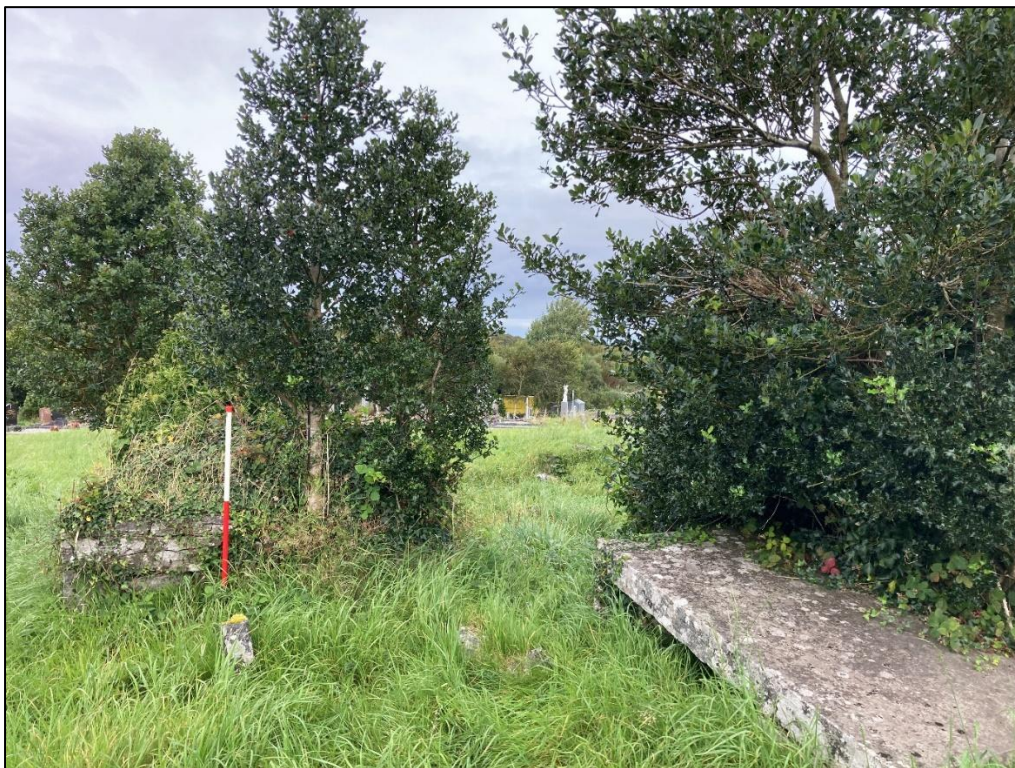
Plate 36: South elevation of nave, west end, masonry has mostly been lost. Appears to have been original point of entry according to 1839 description (see section 4.2.3).
